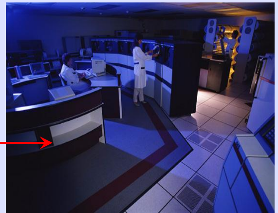
Utility Host Itron/UTS MV-90 Computer Automated Dial-out Meter Reading System
